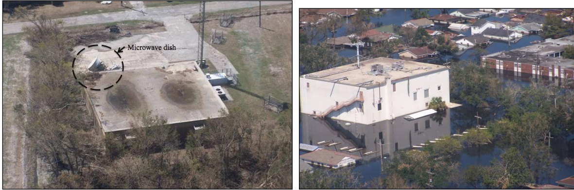
Figure 39. Microwave dish blown off the tower mount (left); flooded central office (right). (Kwasinski, 2006; public domain images)
