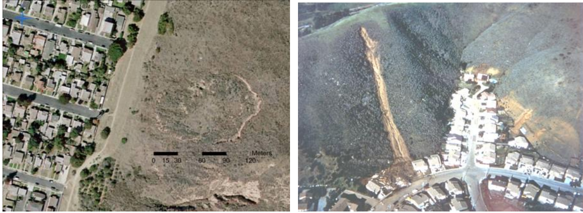
Figure 16. Deep-seated landslide in Ventura Calif., January 2005 (left, photo credit: J. Stock, USGS), and 1982 debris flow in Pacifica, Calif., that killed 3 (right, photo courtesy of Woodward Clyde Consultants).
